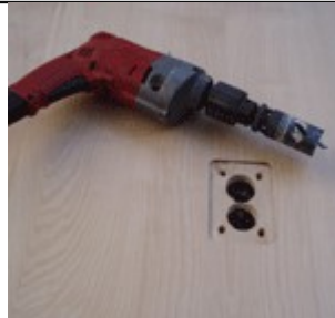
Use a 1 & 3/8" hole saw to drill out the two center holes
