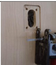
Use a Jigsaw to cut out the wood between the two center holes.
